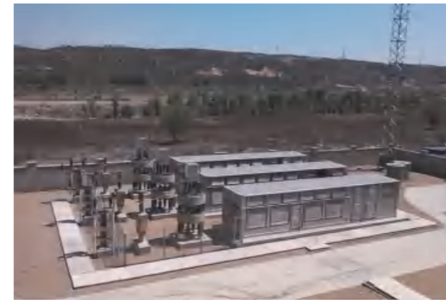
Photos of project on site 1
