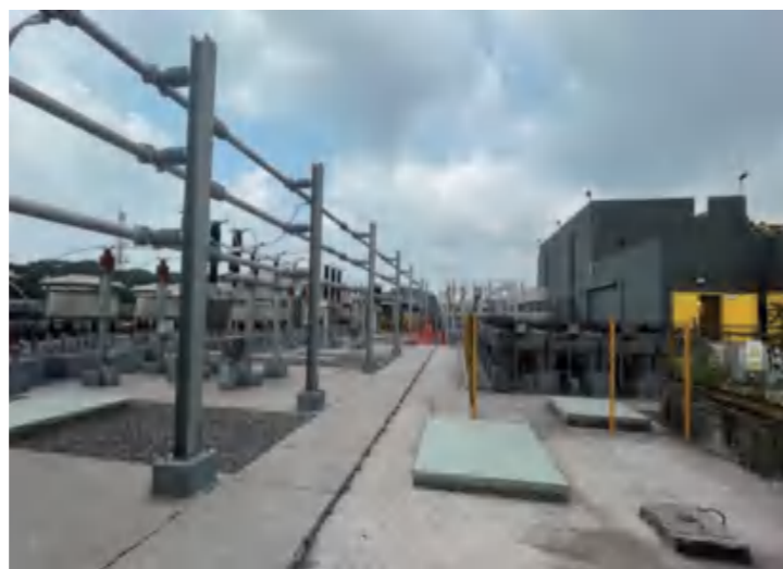
Photos of project on site after installation
