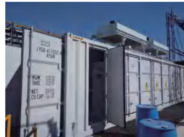
Photos of project on site 2
