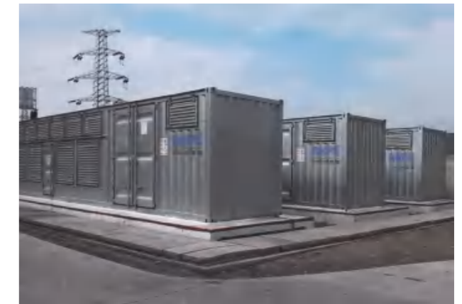
Photos of project on site 2
