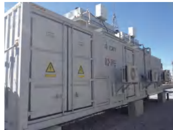
Photos of project on site 1
